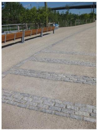
**Figure E. 5:** In-grade textured surfacing, in this case cobble rumble strips
